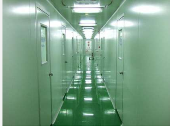
GMP standard purification workshop
