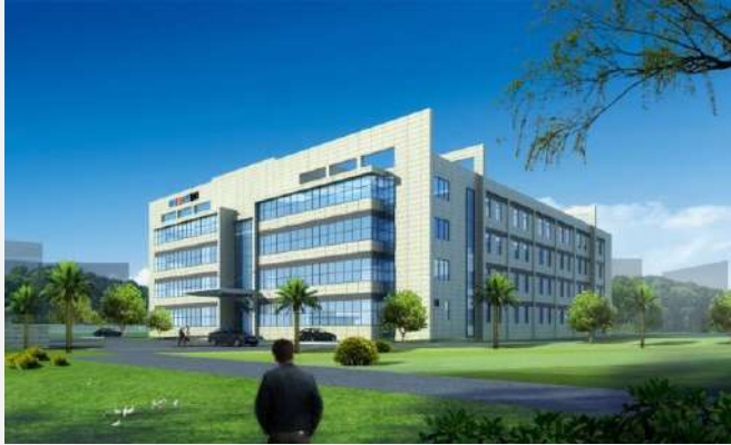
15,000 square meters industrial park
